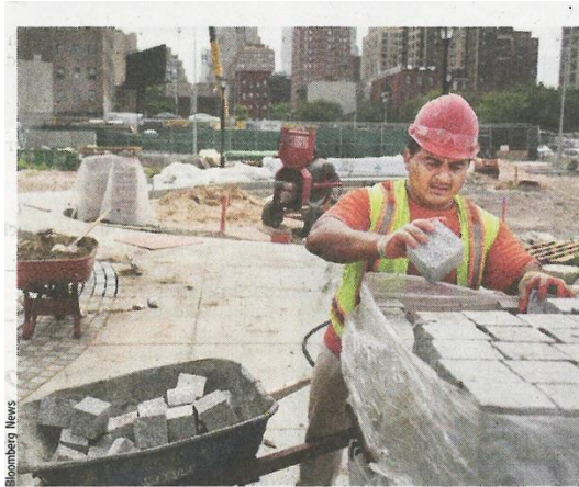
Construction workers at Hudson Yards on Manhattan's far West Side.
